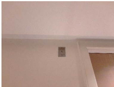
fire alarm indicator lamp
