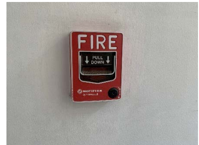
fire alarm manual station
